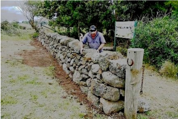
Phil Lane repairing Yatmerone's stone wall
